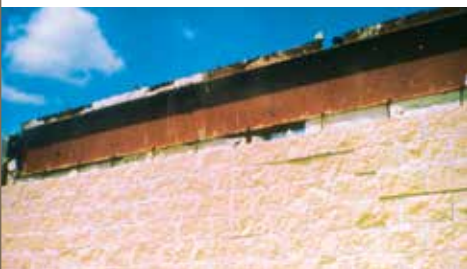
An inadequately designed parapet wall with masonry blocks was blown off at the roof line.
